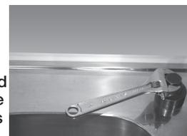
**Step A** – Drill a ¼" pilot hole. Use a ½" Hole Punch and an adjustable wrench to punch the hole in the sink.
