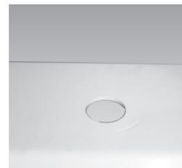
**Step D** – Make sure the surroundings of the sink are cooled before mounting the faucet to the sink after drilling and remove all sharp edges.
