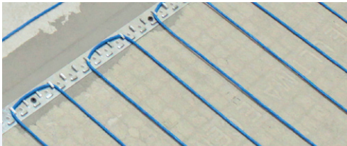
WarmWire installed using CableStrap
